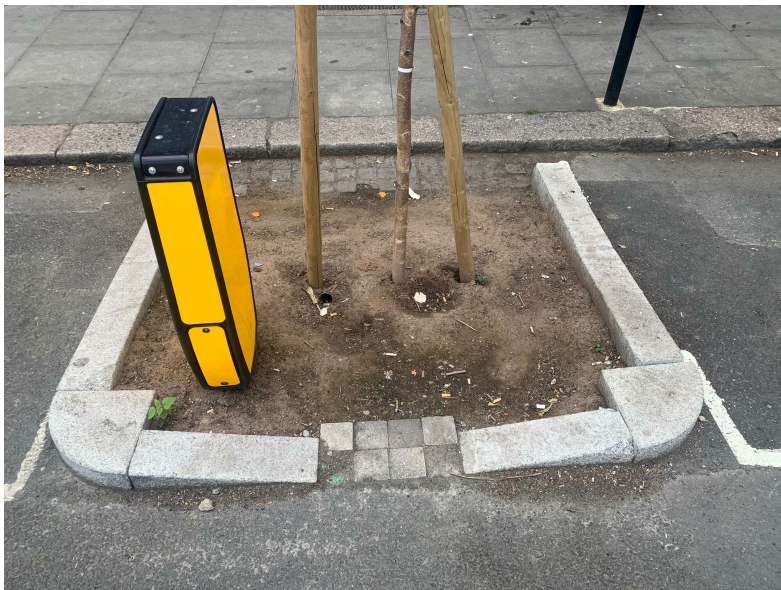
Fig 4. Gulleys draining rain water from the streets to be directed into the tree pit, Kentish Town, Camden Council
