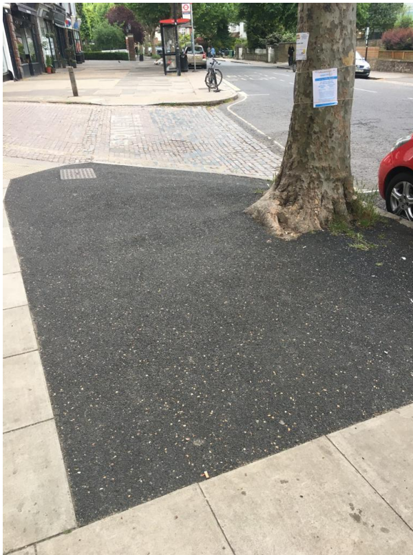
Fig 4. Highgate, Swain's Lane, Permeable tarmac.
